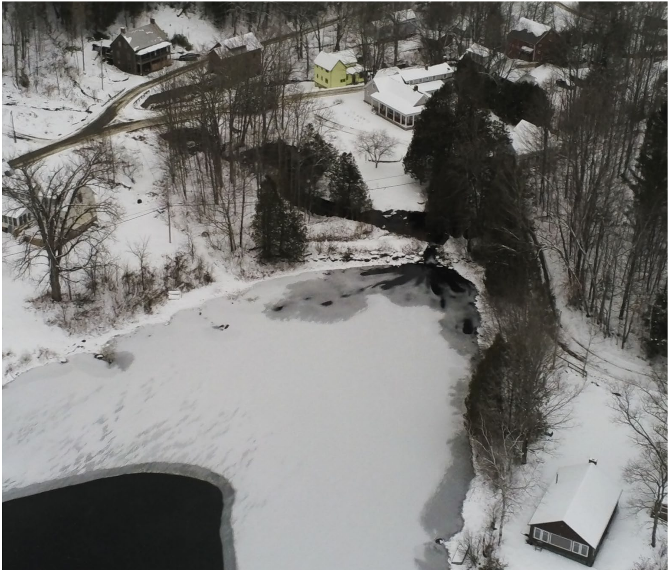
Figure 13: Mirror Lake Dam in Calais
