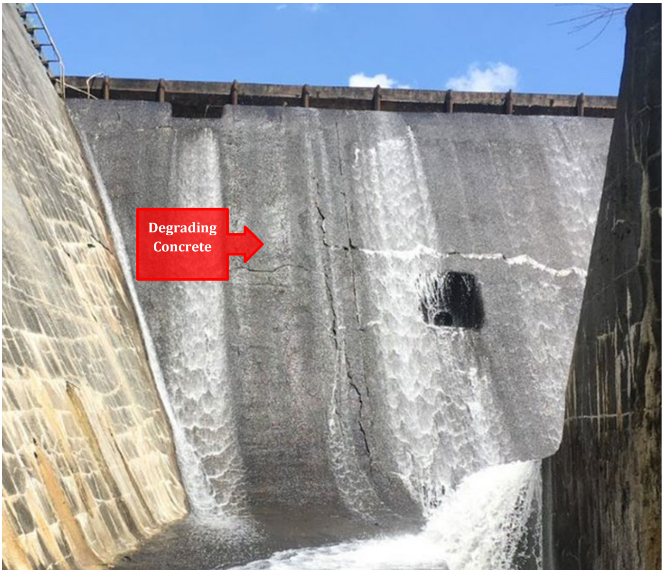
Figure 5: Degraded Spillway in the Thurman W. Dix Reservoir Dam in Orange, Vermont
